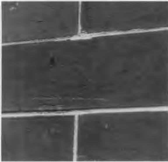
Figure 3. Good-quality repointing closely replicates the original in composition, texture, joint type and profile on this 19th century brick building (left), and on this late-19th century granite on H.H. Richardson's Glessner House in Chicago (right). Photos: Charles E. Fisher; Sharon C. Park, FAIA.
