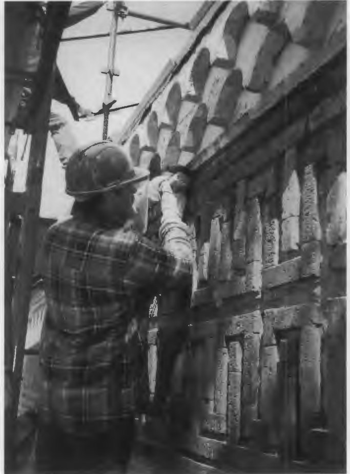
Figure 12.. A power grinder, operated correctly by a skilled mason may be used in preparation for repointing to cut wide, horizontal mortar joints, typical of many early-20th century brick structures without causing damage to the brick. Note the use of protective safety equipment. Photo: Robert C. Mack, FAIA.
